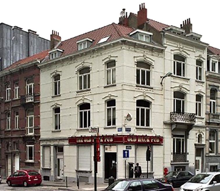
To the left of the white building, the Ecumenical Centre in Brussels housed MPG's first office
