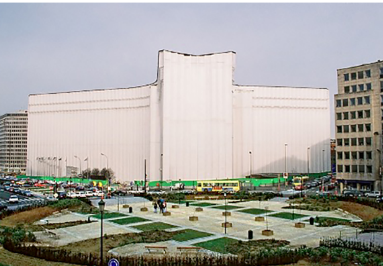
Across the street from MPG's office was the Berlaymont Building, the seat of the EU Commission. It took 13 years to renovate the building, including the removal of asbestos, for which it was hidden behind a white protective screen.
